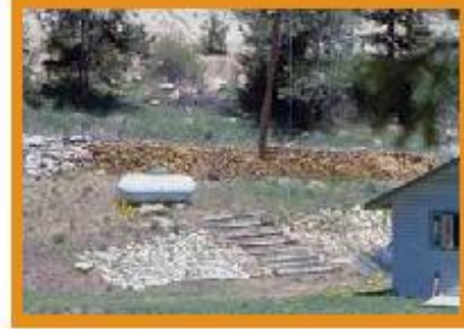
Figure 19: Keep firewood, propane tanks and natural gas meters at least 30 feet away from structures. Photo: CSFS
