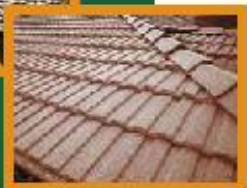
Figure 9: (above right) Class A roofing materials including tile, clay, concrete, slate and asphalt shingles are fire-resistant options. Photo: CSFS
